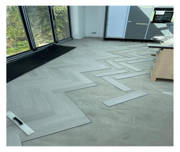
The most important thing to do when installing the herringbone is to use the plastic or nylon headed mallet to fully tap down the ends which is shown in the short video <u>INSTALLING</u> <u>IMPERVIA HERRINGBONE</u>. This is the most crucial part of the installation to ensure everything is locked together. Do not hesitate to bang hard as you will not damage the surface.
