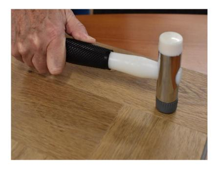
Make sure you use a plastic or nylon hammer to give sufficient "shock" to the ends to fully lock the piece together. You must do this before going on to the next. If you fell it is not locking properly then it is probably down to not fully push fitting the piece into the groove of the locking profile. The image below shows an actual installation of the herringbone by one of our trade clients
